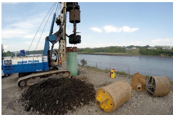
Figure 5 Site of Preliminary Test pile
