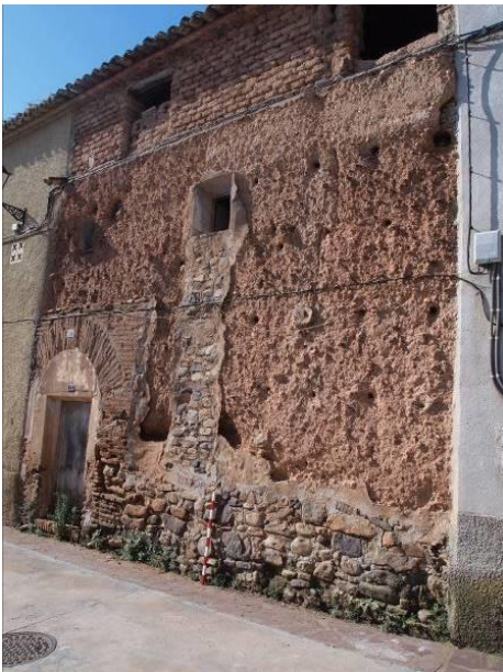
Figure 3: RE house displaying mild coving due to rising damp despite stone base, Ambel.
