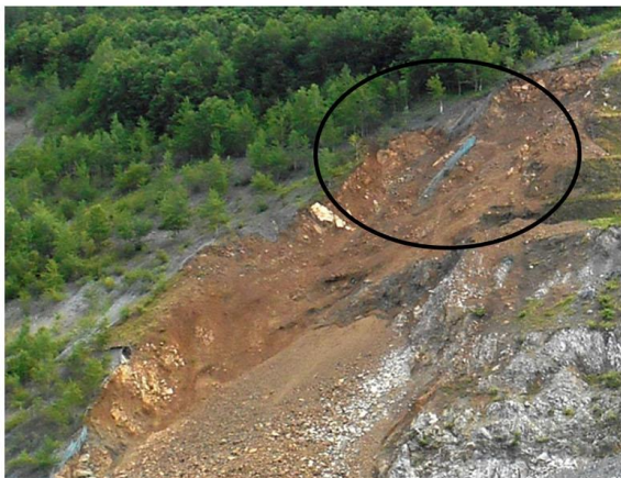
(b) after slope failure
