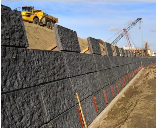
Figure 4. Fake and true horizontal joint alignment.
