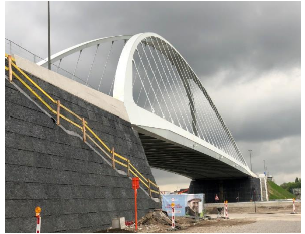
Figure 8. Cladding completed after the bridge placement.
