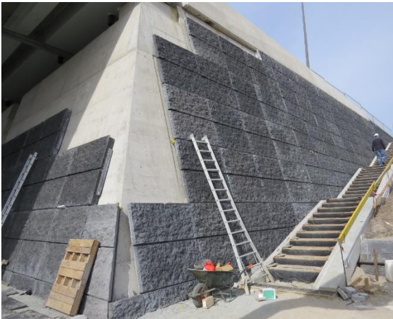
Figure 7. Retaining walls completed, cladding installation.
