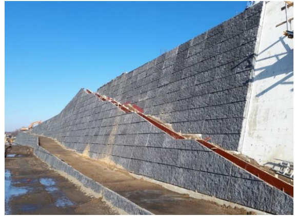
Figure 3. Cut top panels according to architects' requirements
