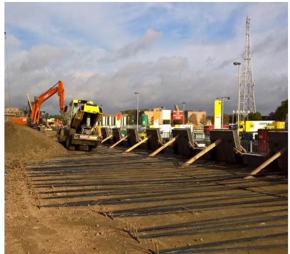
Figure 6. Soil placement and compaction.
