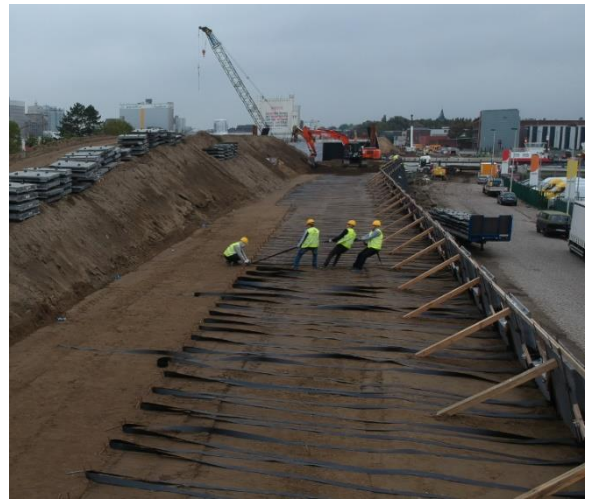
Figure 5. ParaWeb strips installation.
