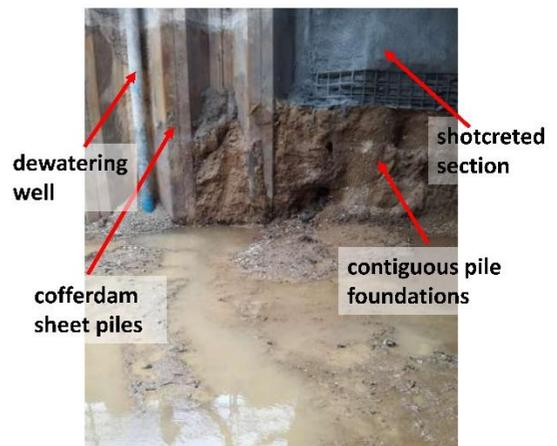
Figure 4. Water ingress at sheet pile and overbridge contiguous piled foundation interface.
