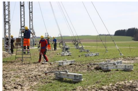
Figure 4. Combination of Spinnankers for anchoring guy wires of temporary line towers, Austria (2018)
