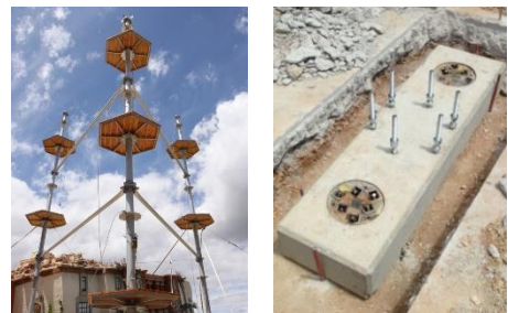
Figure 5. Hybrid foundation of precast concrete and Spinnankers for a climb parc in Spain
