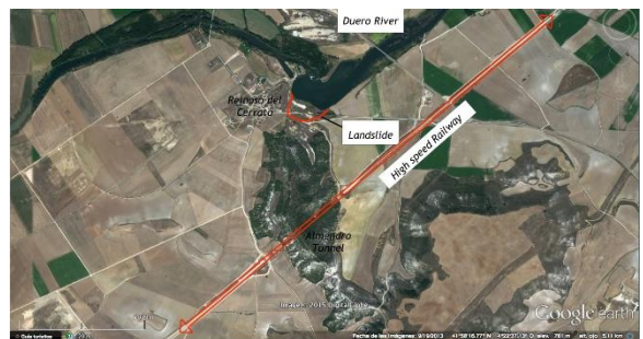
Figure 1. Location of the tunnel (S Reinoso, Palencia)
