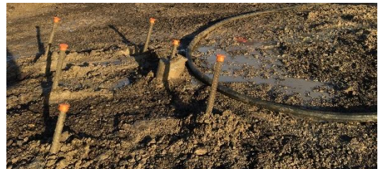
Figure 2: Micropiles installed at a rake of \sim 15^\circ
