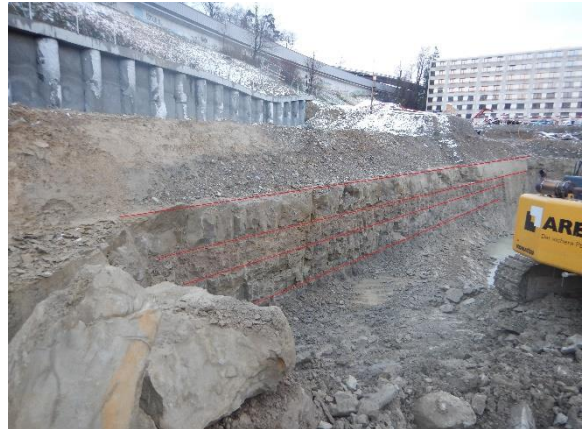
Figure 4. Molassic rock with different layers and different degrees of alteration (indicated by red lines)
