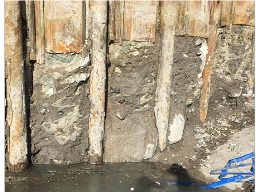
Figure 1 Photo's above show example evidence of local buckling of steel sheet pile toes, two photo's below show unearthed toe of sheet pile wall. Photo: P. Björgúlfsson & K. Viking.
