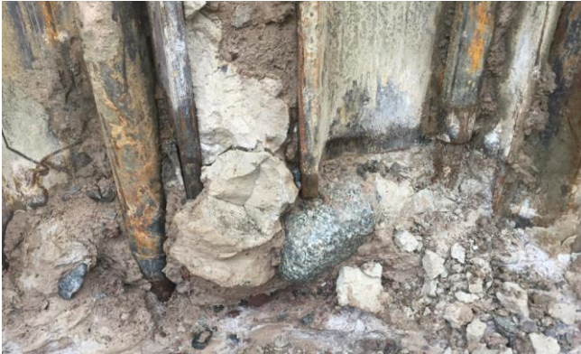
Figure 1 Photo's above show example evidence of local buckling of steel sheet pile toes, two photo's below show unearthed toe of sheet pile wall. Photo: P. Björgúlfsson & K. Viking.
