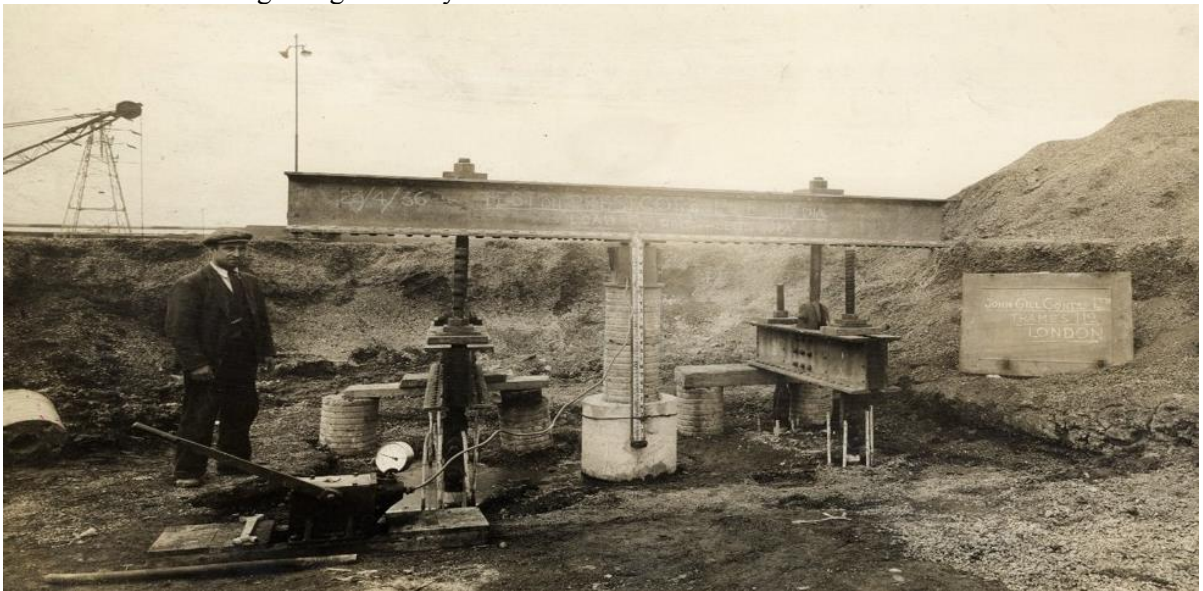
Figure 1. A compression load test carried out in Yorkshire, UK. 1936.
