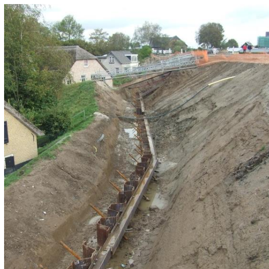
Figure 1: Installation of discontinuous sheet pile wall as reinforcement of Lekdijk Krimpenerwaard
