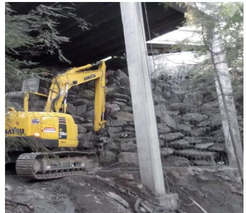
Figure 9: Slope stabilisation under a newly built residential car park. No damages were observed during and after the earthquake. The potential damage of slope failure would have resulted in the collapse of the residential compound and the car park.
