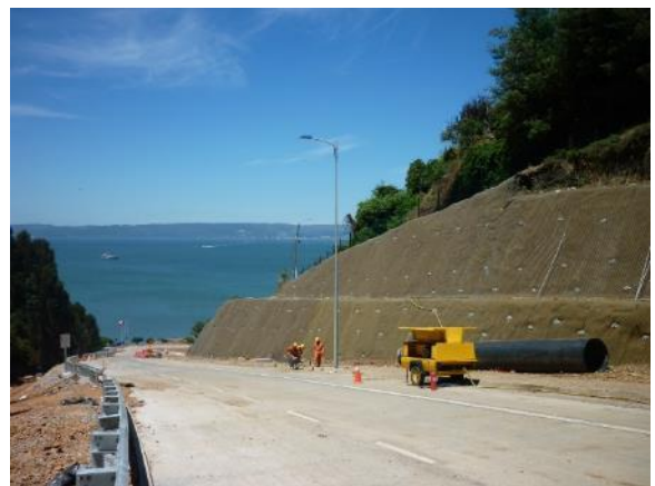
Figure 13: Overview of the stabilised road stretch being. No deformation or failure after the earthquake.
