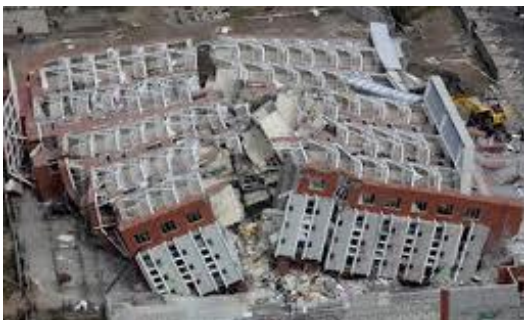
Figure 11: Damage in Caleta Tumbes, Talcahuano after the earthquake.
