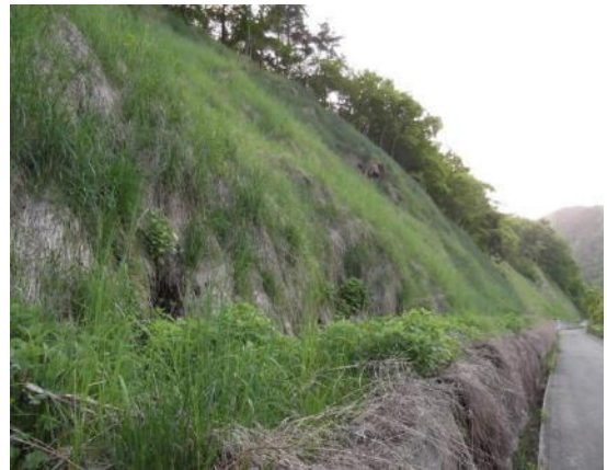
Figure 6: Not far away, a stretch of road where the slope stabilization was done with high tensile steel flexible system and soil nailing and has long been re-vegetated, in Tono City. The whole stretch of slope along the road remained stable throughout the earthquake swarm.
