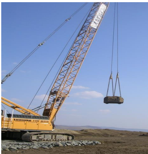
Figure 4. Dynamic compaction
