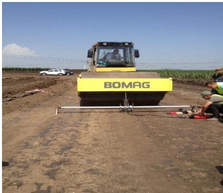
Fig. 10 In-situ verification of bearing capacity with Lucas plate
