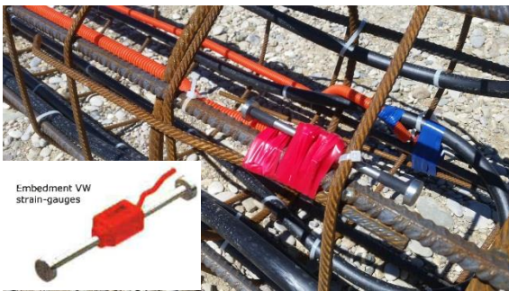
Figure 10. Strain gauge sensor installation
