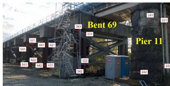
Figure 11. Typical monitoring points
