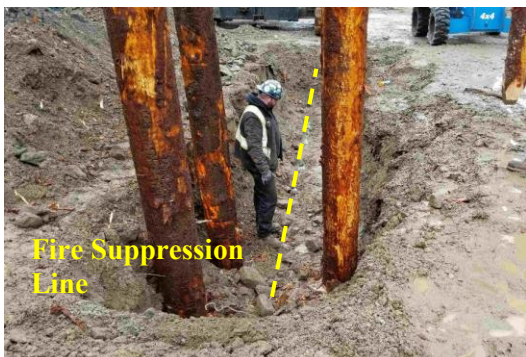
Figure 10. Pile driving adjacent to utilities
