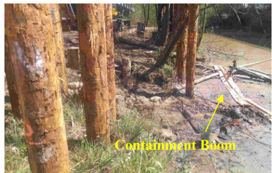
Figure 9. Pile driving adjacent to the river bank
