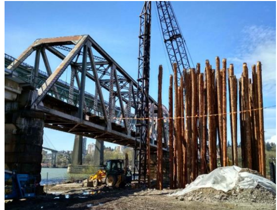
Figure 8. Pile driving adjacent to railway track
