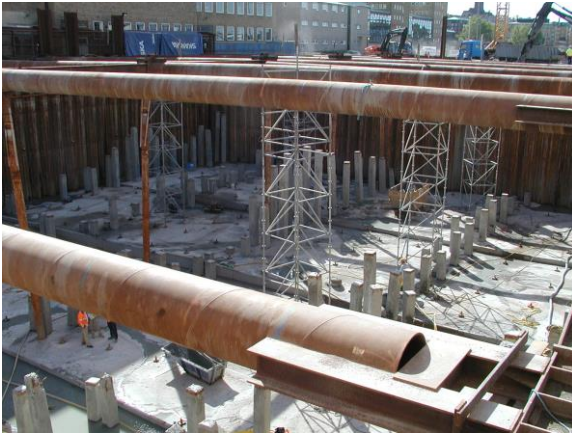
Figure 3. Excavation after dewatering.
