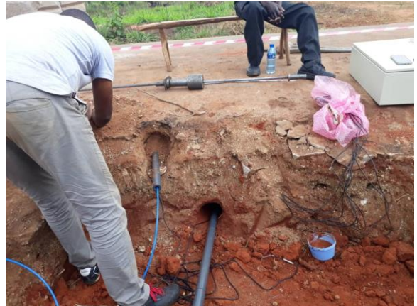
Figure 10. The study road in Tanzania and the installation devices
