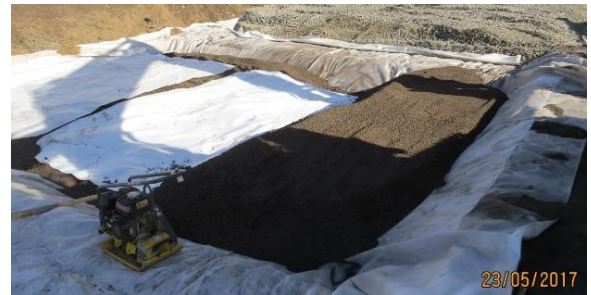
Figure 7 Construction of the basin (wrap-around structure in the front). The geotextile is pulled over on top of the LWA layer. (Photo: S. Frimodig 05/2017)
