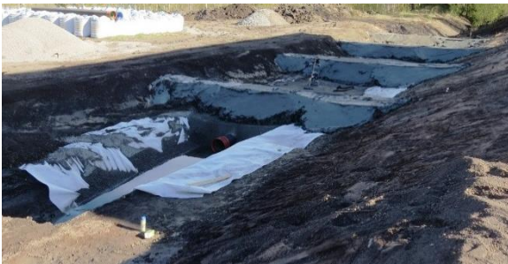
Figure 3 Complete clay basins before LWA fill. The size of one basin is 6.5 m x 7 m (Photo: S. Frimodig 05/2017)
