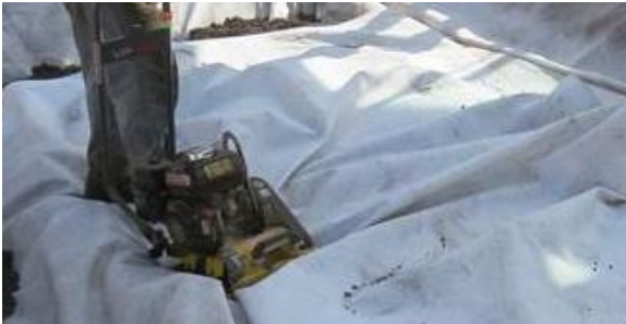
Figure 6 Compaction method tested in wrap-around structure 3. (Photo: S. Frimodig 05/2017)
