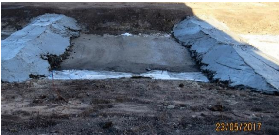
Figure 4 One of the testing sections before LWA fill. (Photo: S. Frimodig 05/2017)
