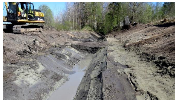
Figure 1 Forming the surface of clay and excavating the pipeline trench before construction of the test structures. (Photo: S. Frimodig 05/2017)
