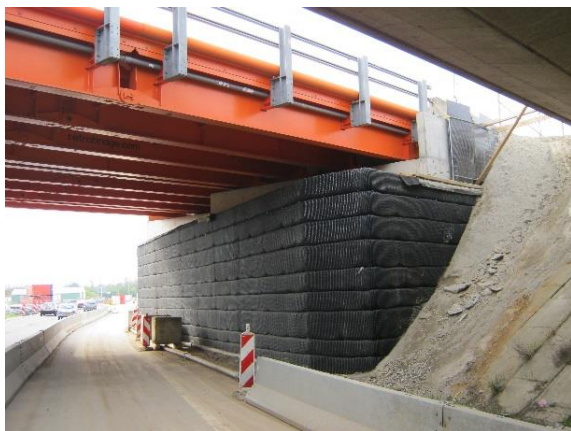
Figure 3. GRS wall as highly loaded temporary bridge abutment
