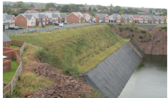
Figure 2. GRS wall after vegetation
