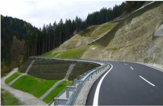
Figure 14. Constructed GRS walls
