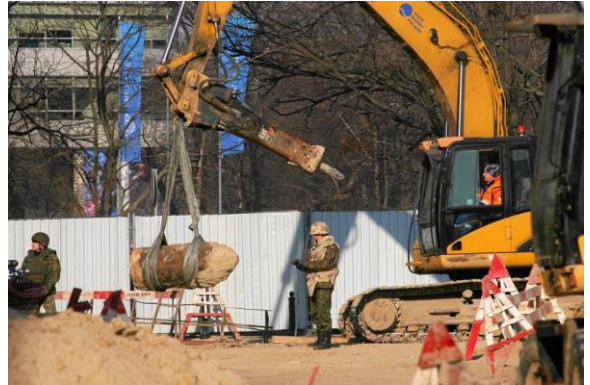
Figure 1. Karl missile discovered in the excavation
