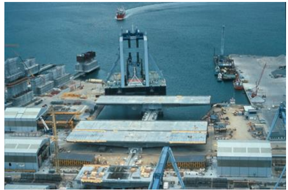
Figure 9. Lindholm pre-fabrication yard for the West Bridge deck and pier elements
