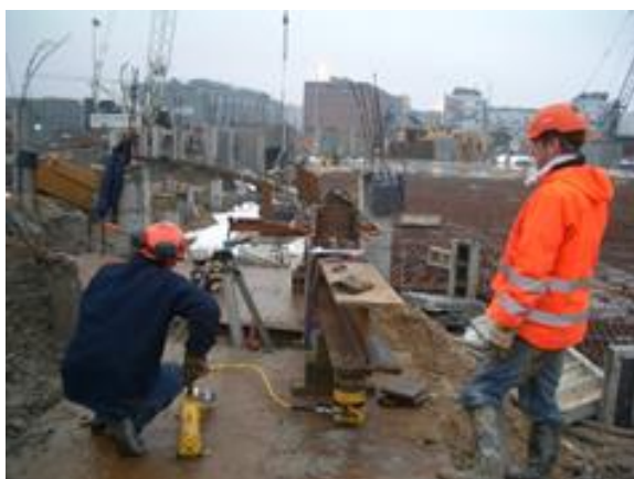
Figure 6. Tension pile testing at Sluseholmen
