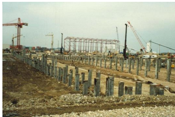
Figure 7. Piles for sliding ramp, Nordhavn
