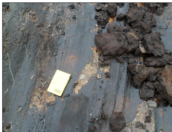
Figure 6. Black hard pan below failed peat (F2)
