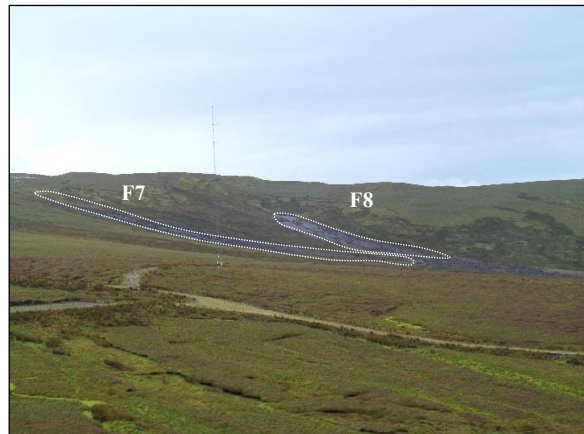
Figure 5 General view of landslides F7 to F8)
