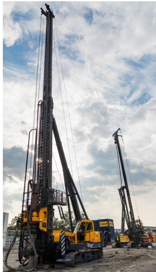
Figure 8. Installation of FDP 40m test pile
