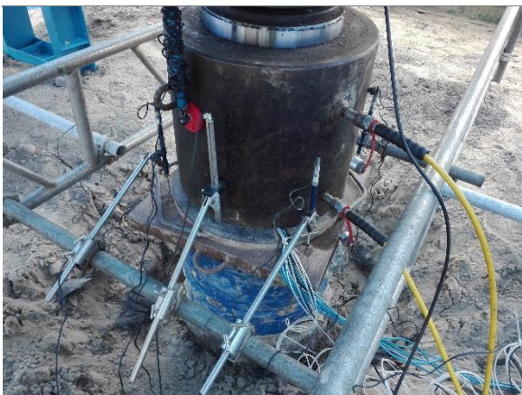
Figure 7. Instrumented pile head during SLT
