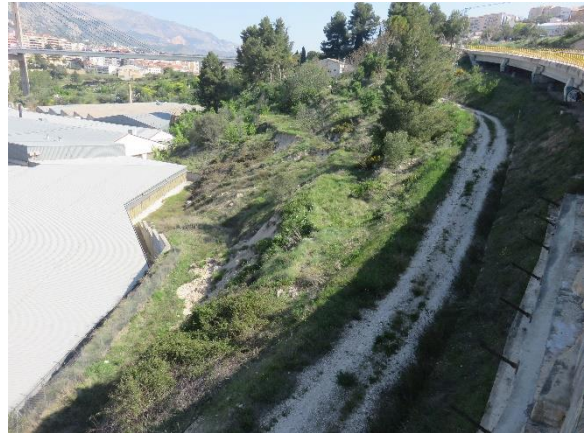
Figure 3. General view of the slope.
