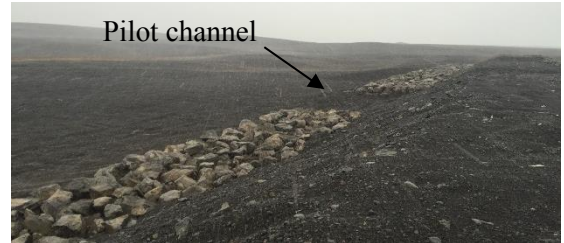
Figure 6. Fuse plug in Svartárstífla dam. View of the pilot channel, downstream.
