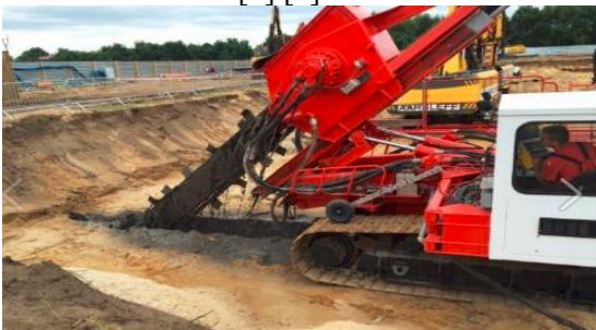
Figure 4 Trencher used in Trechmix technology
