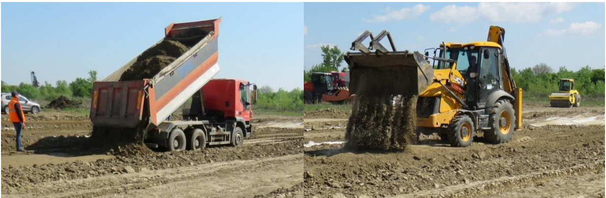
Figure 6. Spreading of the clayey soil and sand in addition
