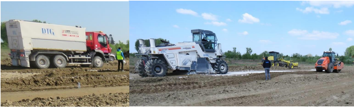
Figure 7. Spreading of 2.5% hydraulic binder, mixing of the si.Cl with the hydraulic binder and the compaction with the cam roller
