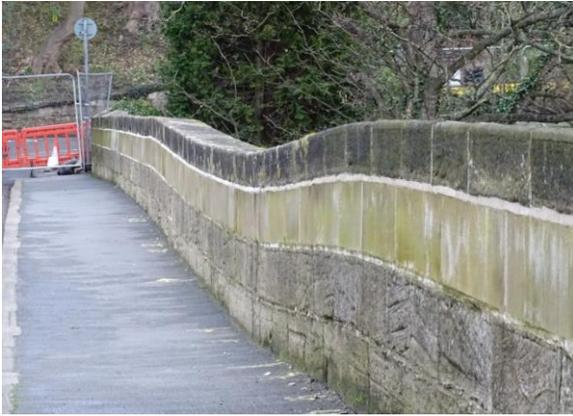
Figure 3. Sunken parapet above the south pier
