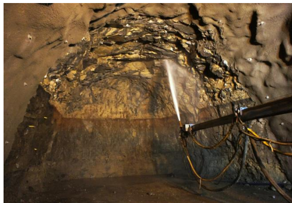
Figure 10. Mixed face, columnar basalt overlaying, sedimentary rock, st~2.200
