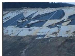
Figure 3. Example 3 – closing of an old landfill – improper design of the side slopes without geotechnical calculations
