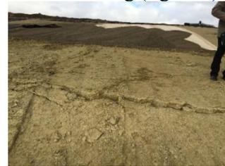
Figure 9. Case study – old landfill – fissures appeared during the capping works – slope
