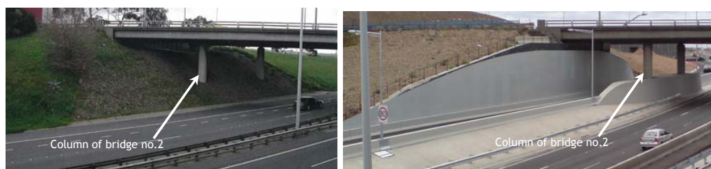
Figure 2: The site prior to and after completion of works for the Bulla Road exit ramp
