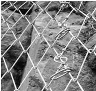
Figure 3. T3 Clip used to connect TECCO® panels vertically in rock (left) and in soil application (right).
