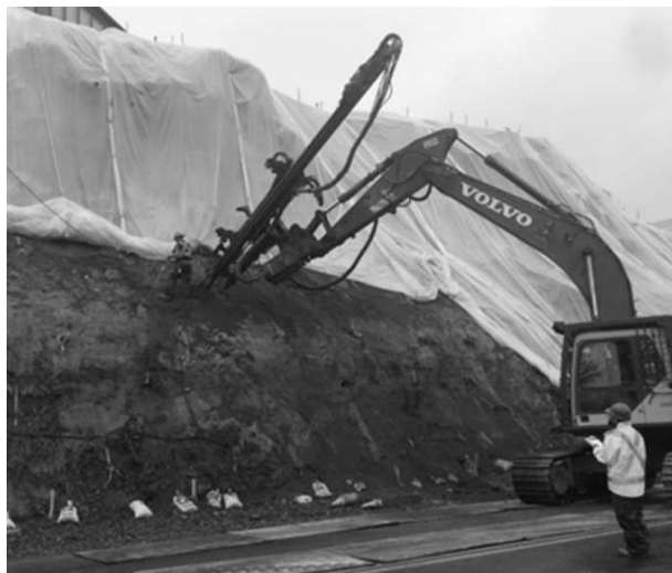
Figure 9. Installation of soil nails with excavator.
