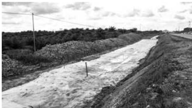
Figure 5. Laying out Geotextile complete
