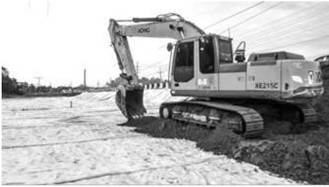
Figure 6. Backfill soil and compaction.
