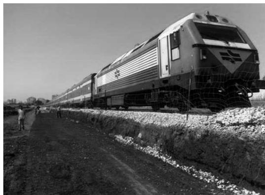
Figure 4. Due to the shallow excavation for the thinner geocell solution no support is needed for the adjacent track under operation
