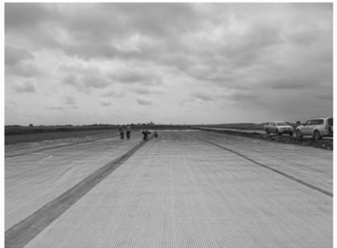
Figure 2. Right hand side of trial embankment, installation of geocomposite (Fortex 35/35+ geotextile)
