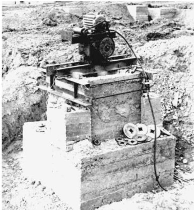
Figure 10. Dynamic testing of a production pile foundation on 4 precast reinforced piles C10-30, 10 m long.
