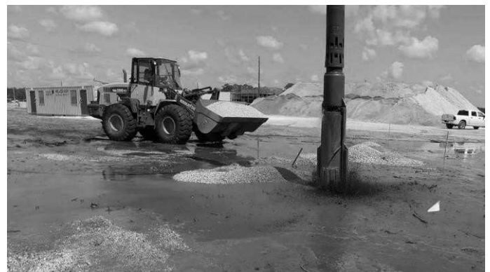
Figure 6. Stone column installation Table
