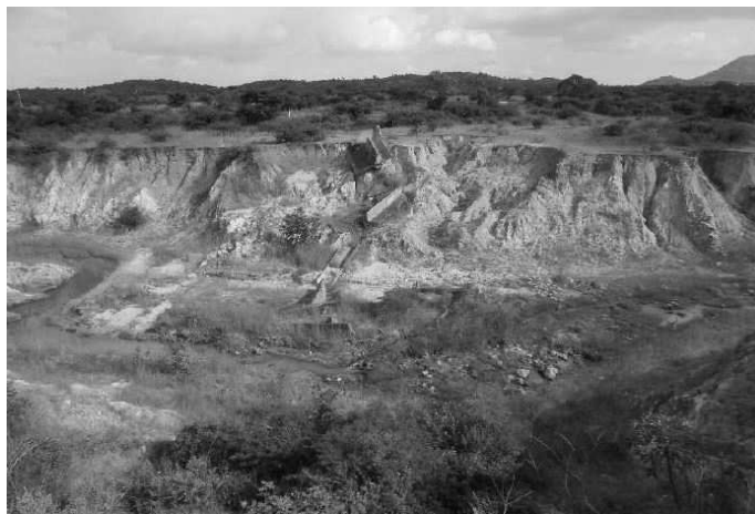
Figure 1. View of donga at old spillway section
