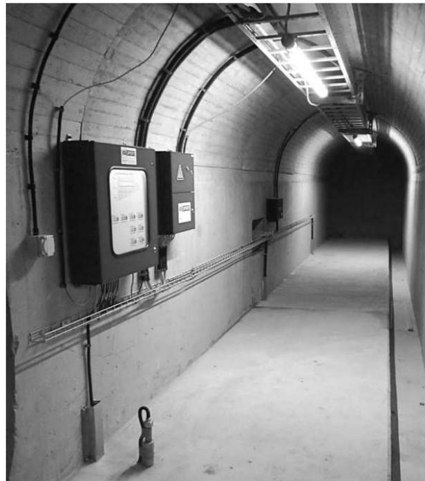
Figure 11. Measuring box for the flotation measurements with digital displays of the current heads
