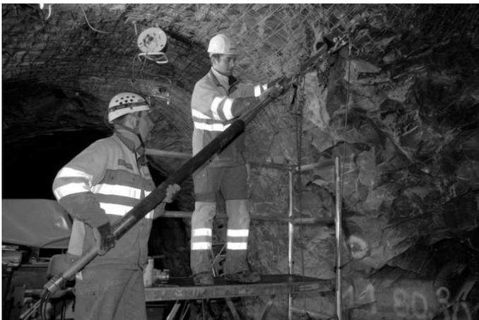
Figure 3. Installation of the multi-packer system
