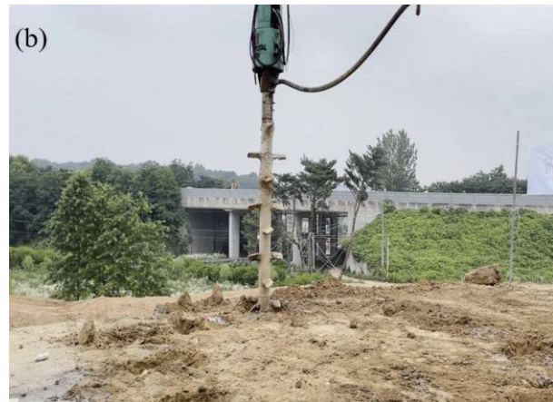
Fig. 1 Field tests conducted on Zian Co. Ltd. Headquarters at Boryeong, Chungnam, South Korea (a) layout of WAB stabilized soil columns at testing site; and (b) picture of actual installation of soil columns with WAB
