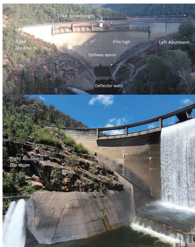
Fig. 2. Bendora Dam configuration with close-up of right abutment
