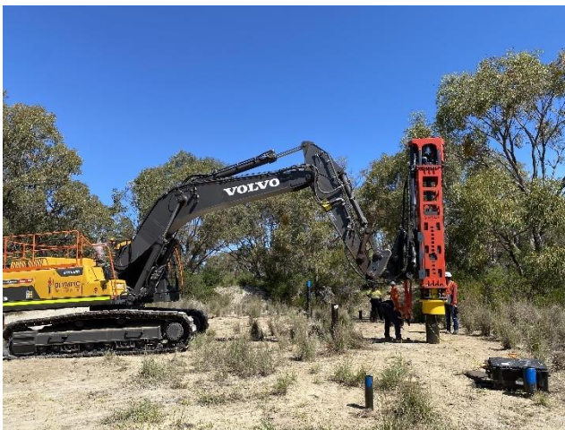
Figure 3. Pile installation in variably cemented carbonate sand.
