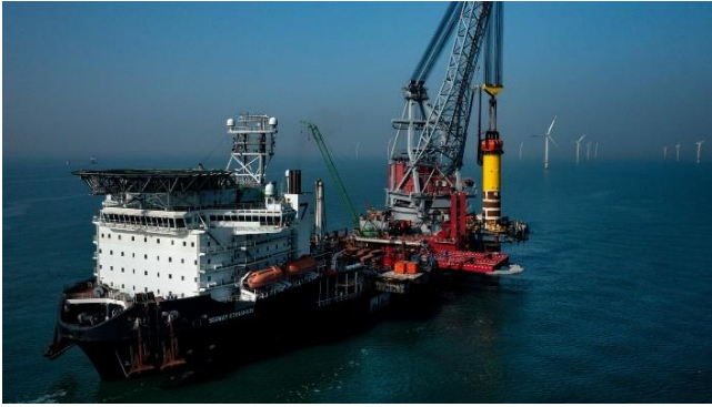
Figure 1. Vibro-driven monopile installation (source: Cape Holland).
