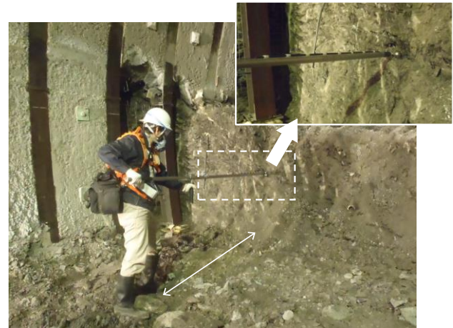
Figure 5. The implementation status of KBI in tunnel faces.
