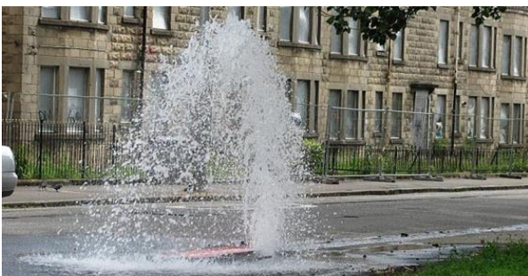
Figure 1 Underground freshwater leakage image (Water matters UK2013).
