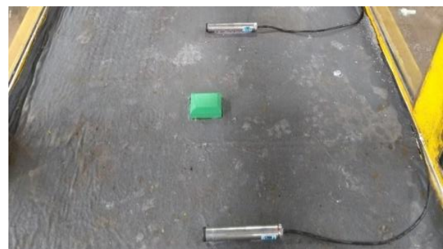
Figure 3 - Installation of piezometers and base of optical inclinometer
