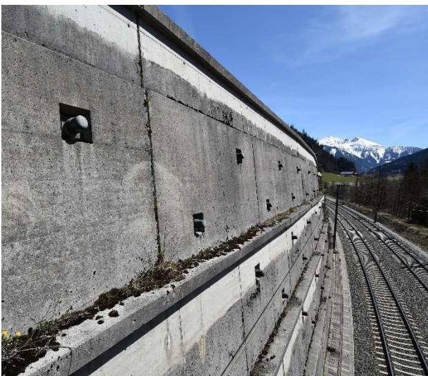
Figure 1: Anchored structure in Austria.
