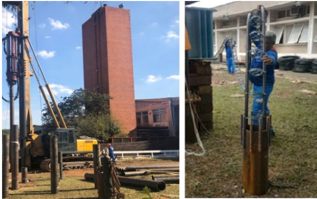
Figure 1. Steel pipe energy pile installation at the University of São Paulo (de Freitas Murari et al., 2022).
