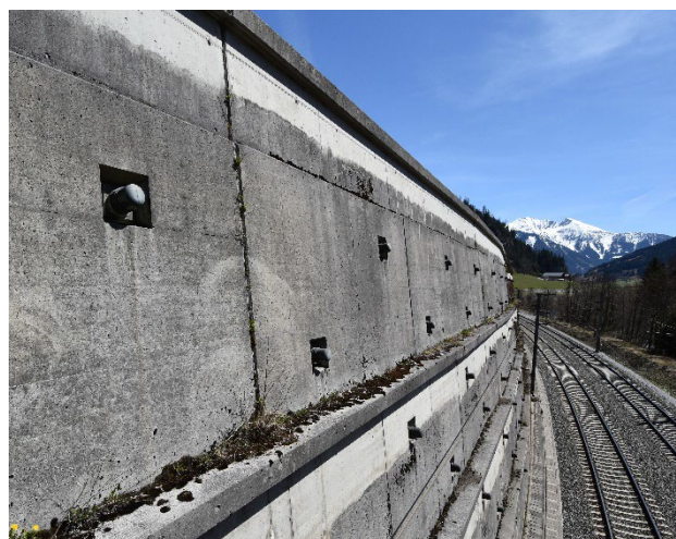
Figure 1. Example of an anchored structure along the railway network in Austria.
